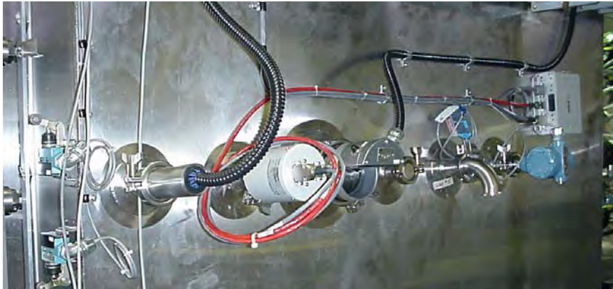
Pressure and Vacuum sensors mounted on Triclover connections
